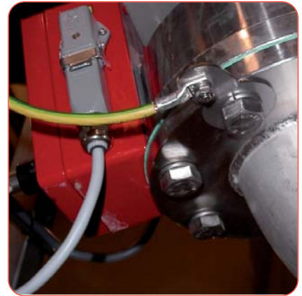
HF-Ground connection AIS-Suppressor
